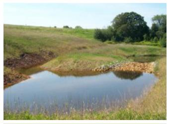
**Forebay at De Sale Phase 3:** The forebay at the De Sale Phase 3 passive treatment system intercepts AMD from reclaimed mine spoil and helps to settle suspended solids and collect iron-bearing precipitates.
