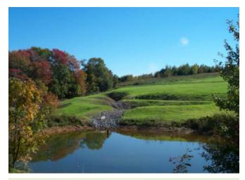
**Phase 3 Settling Pond:** A pond that was formerly part of a chemical treatment facility was repurposed as a settling pond (foreground) at De Sale Phase 3. This settling pond receives effluent from a vertical-flow pond and helps remove and store suspended solids and debris.
