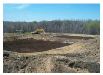
**Compost in Vertical-Flow Pond:** About 6 inches of spent mushroom compost is placed atop limestone in vertical-flow ponds.
