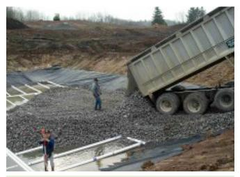
**Vertical-Flow Pond Construction:** Limestone aggregate was used in the construction of flushable, vertical-flow ponds. The limestone, topped with spent mushroom compost, neutralizes acidity, raises pH, and removes metals from the effluent.
