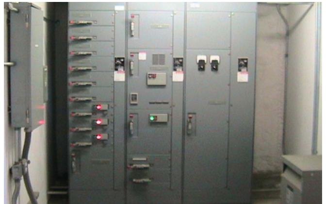
Integrated Electrical Controls: The site's PV-generated electricity supplements grid-supplied electricity consumed at the treatment plant.
