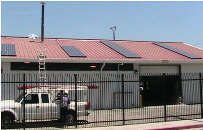
PV Panel Installation: The PV system consists of 20 panels that were installed on the treatment plant roof over four days in June 2007. The south-facing steel roof is approximately 81 feet long and 28 feet wide, with a 4:12 pitch and 20-foot-high ridge. The solar panel collateral load is approximately four pounds per square foot.
