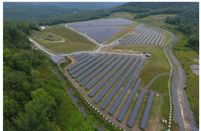
Solar Facility Configuration: The 27-acre solar energy facility is equipped with 19,998 PV panels and three inverters. The inverters convert direct current generated by the PV panels to alternating current, which is sent to a transformer that steps up the voltage for transmission through the local utility lines. Security fencing surrounding the solar farm sits on concrete ballasts to avoid penetration of the waste caps. (photo credit: Conti Solar)
