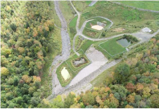
Passive Treatment System Aerial: The passive treatment system relies on the site's existing surface gradients to direct TP-1 leachate sequentially to the anoxic limestone drain, settling pond, vertical flow pond and constructed wetland. The wetland water discharges to Copperas Brook via a cascade that replenishes the water's oxygen content.
