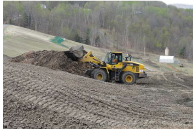
Soil Manufacturing: Onsite manufacturing of organic-rich soil was accomplished through use of machinery fueled with B-20 and equipped with diesel-electric power trains and Tier 4 engines.
