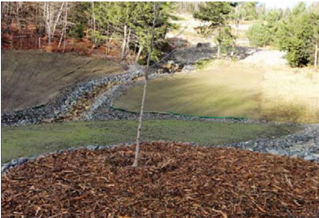
Native Tree Plantings: Native hardwood trees such as red oak and sugar maples were planted along perimeters of the new stormwater retention/detention basins to aid restoration of wildlife habitat and infiltration of rainfall and snowmelt.
