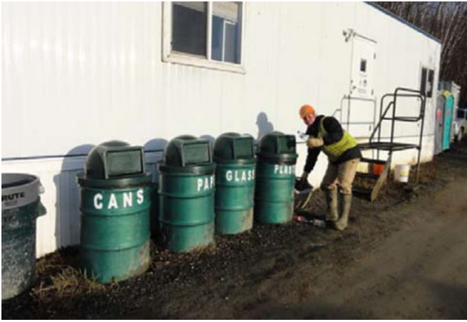
Routine Waste Recycling: Strategic placement of clearly labeled waste containers helped construction workers discard recyclable metal cans, paper, glass, and plastics on a daily basis and streamlined the waste segregation/hauling process.
