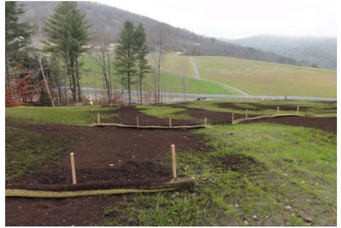
Slope Repair: The blown compost blanket was combined with the tubular sediment-control devices to repair slopes suffering from rills caused by water erosion.
