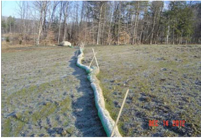
Sediment Control: SiltSoxx™ placed along the TP-1A soil cap perimeter during construction controlled sediment and contained and filtered stormwater runoff prior to its gradual subsurface infiltration.
