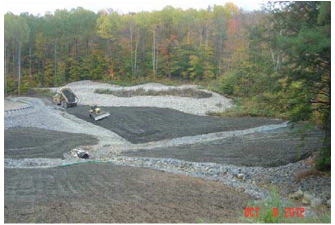
Natural Contours: Designs for backfilling, re-grading, and stabilizing the former sediment basin areas focused on mirroring the site's natural contours and drainage patterns.
