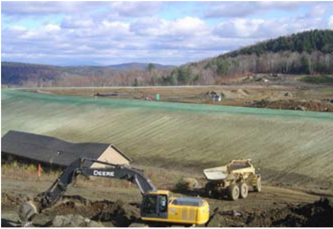
TP-1A Soil Cap: Approximately 380,000 square feet of biodegradable matting was sprayed onto slopes surrounding the TP-1A soil cap.
