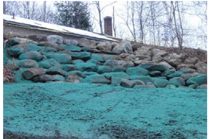
TP-1A Slope Armor: Biodegradable matting and salvaged boulders were used to stabilize restored slopes as needed across TP-1A, including areas adjacent to occupied or abandoned structures.
