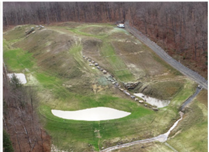
South Mine Before and After: Remedial activity conducted in 2018-2019 at the site's South Mine area, which drains to Lord Brook, included installing a waste cover, converting two former pit lake areas to stormwater retention/detention basins, and constructing a wetland.
