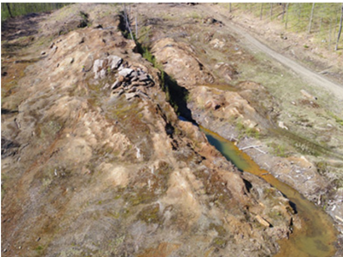
South Mine Before and After: Remedial activity conducted in 2018-2019 at the site's South Mine area, which drains to Lord Brook, included installing a waste cover, converting two former pit lake areas to stormwater retention/detention basins, and constructing a wetland.
