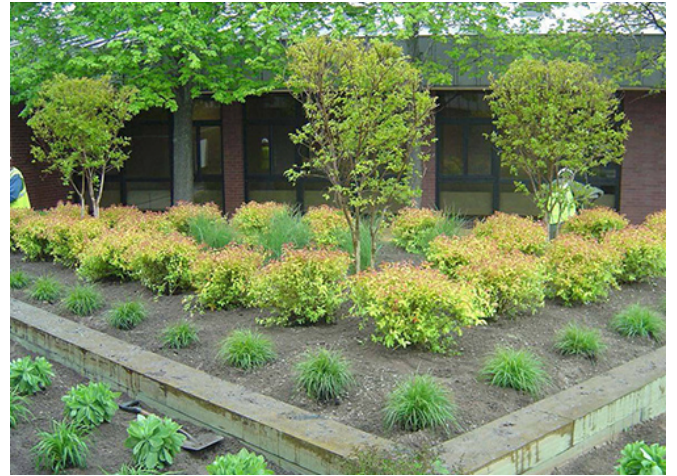
Planter Boxes: Tiered planter boxes with low-maintenance grasses, shrubs and trees that now occupy the former oil burn pit contribute to the site's green infrastructure for capturing and retaining stormwater while enhancing aesthetic features of the site.
