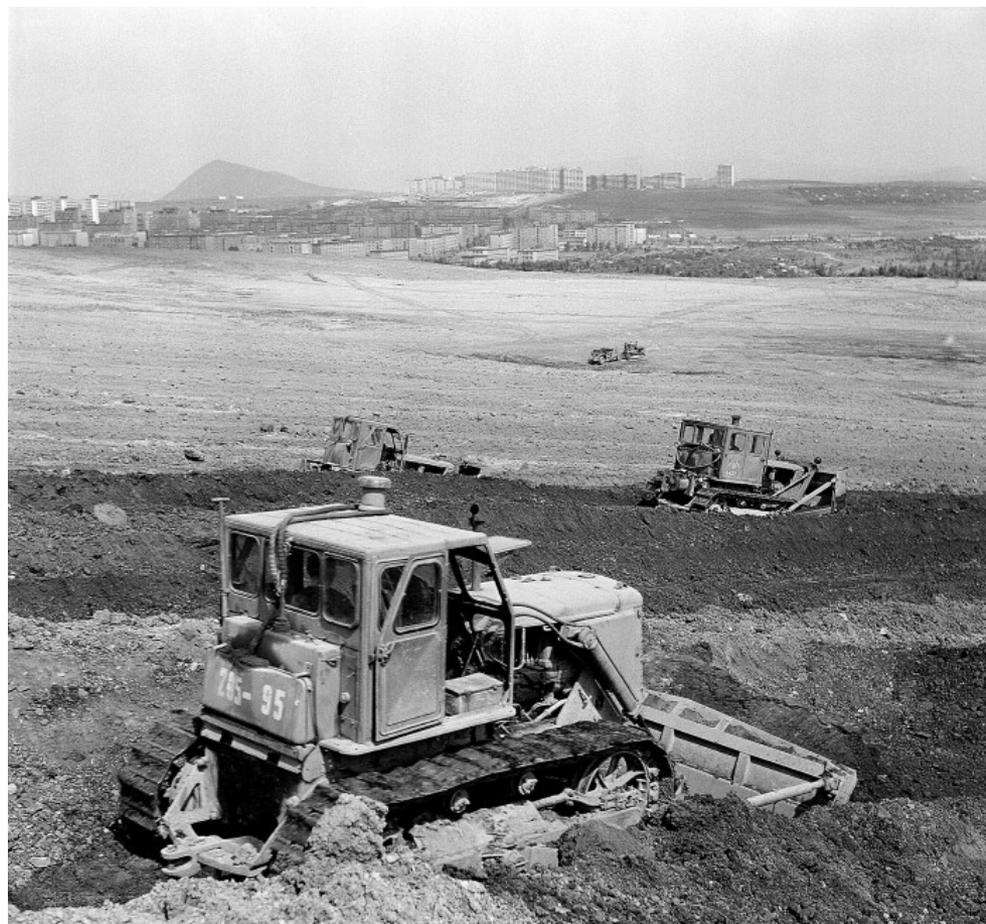
Fig. 3 Outer waste dump beány recultivated to vineyard (1975 and 1975)
