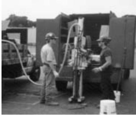
**HRC is injected into the aquifer using direct-push technologies.**
