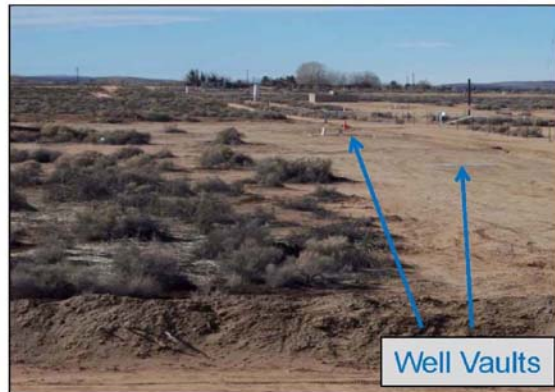
Recirculation well field – wells are below grade within vaults.
