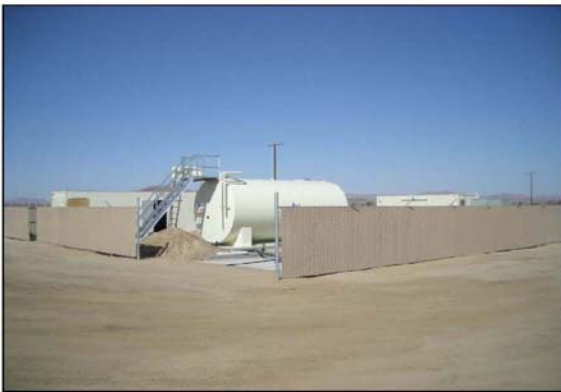
Remediation system buildings and substrate tank matching desert landscape.
