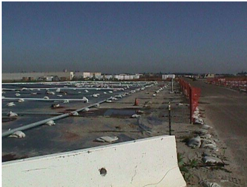
Figure 25. Photograph of IR Site 9 showing plumbing used for SVE system.
