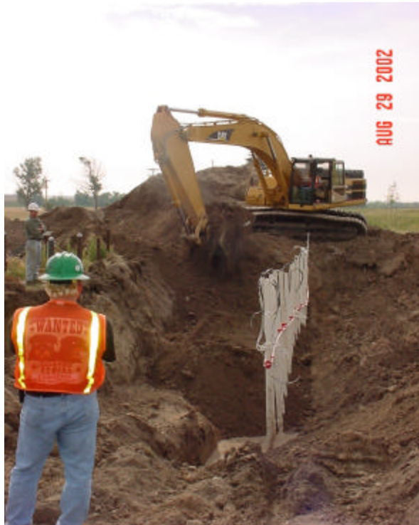
Figure 30. Backfilling of trench with imported soil. Note risers containing electrical connections, gas vests, washout tubing and multilevel sampling bundles
