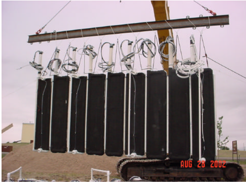
Figure 28. Lifting of nine linked e-barrier modules (panels) prior to placement in trench
