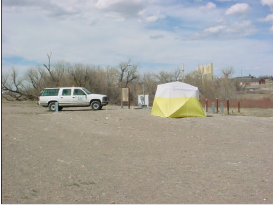
Figure 37. Final grade and sampling shelter
