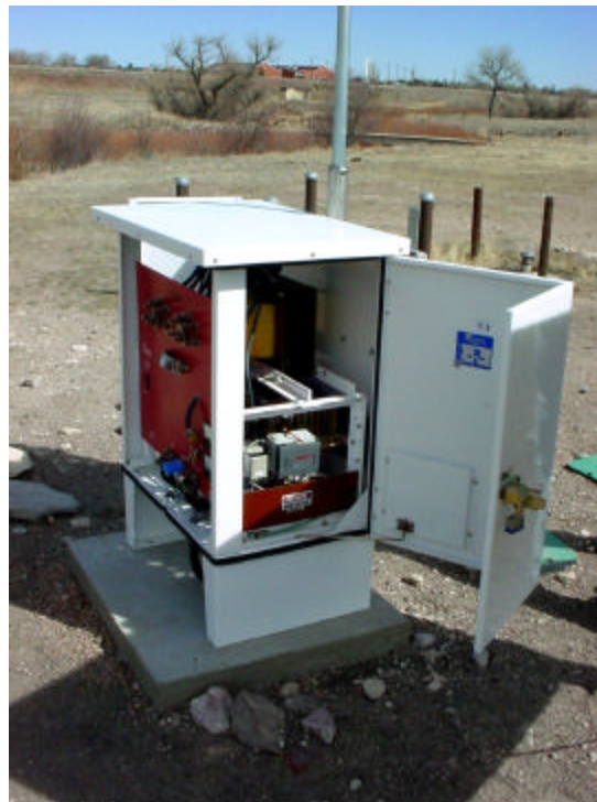
Figure 33. Rectifier and programmable logic controller for electrode reversal (scale management)
