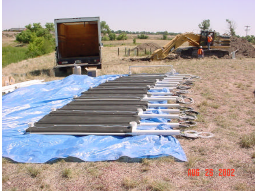
Figure 26. Layout of e-barrier components prior to field assembly
