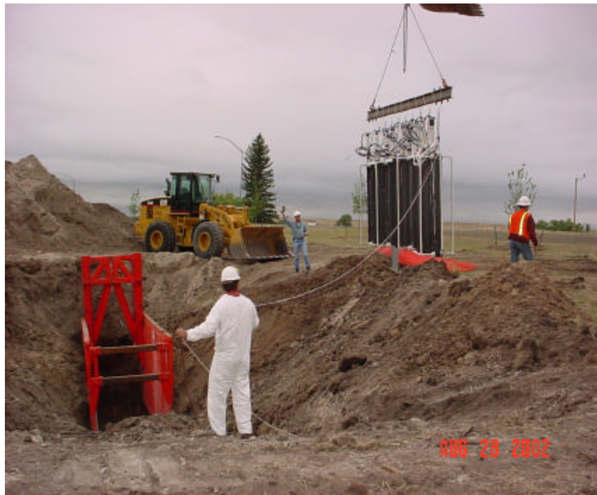
Figure 29. Placement of eight linked e-barrier modules into the trench linking with in-place e-barrier modules
