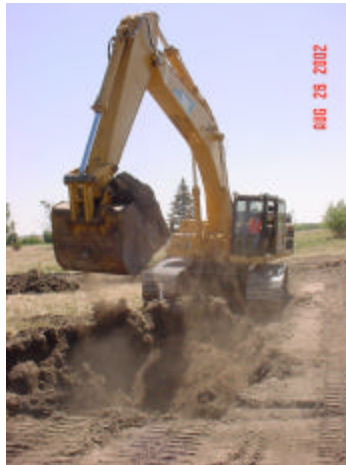
Figure 25. Excavation prior to trench box installation
