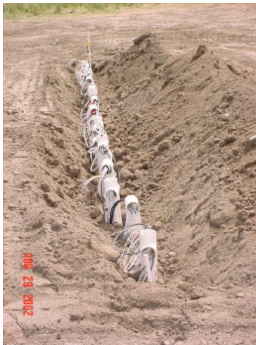
Figure 31. Top of risers prior to surface completion
