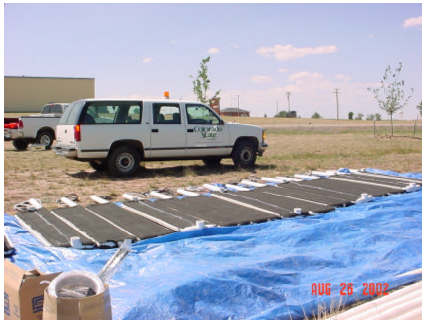
Figure 27. Layout of e-barrier components prior to field assembly
