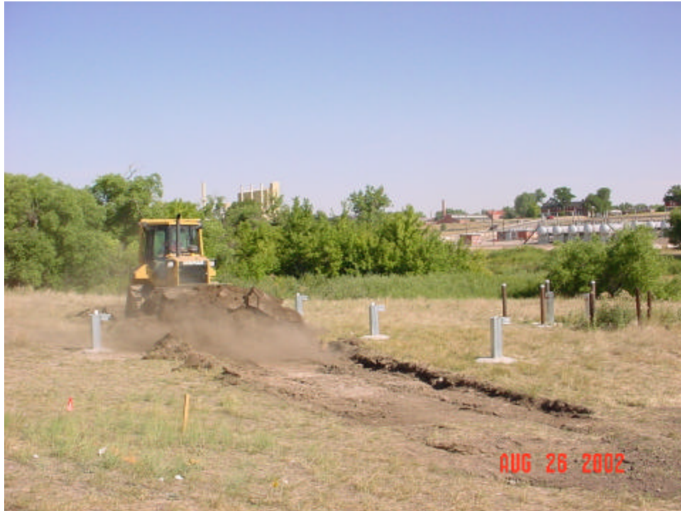
Figure 24. Initial topsoil removal prior to excavation for installation of demonstration e-barrier
