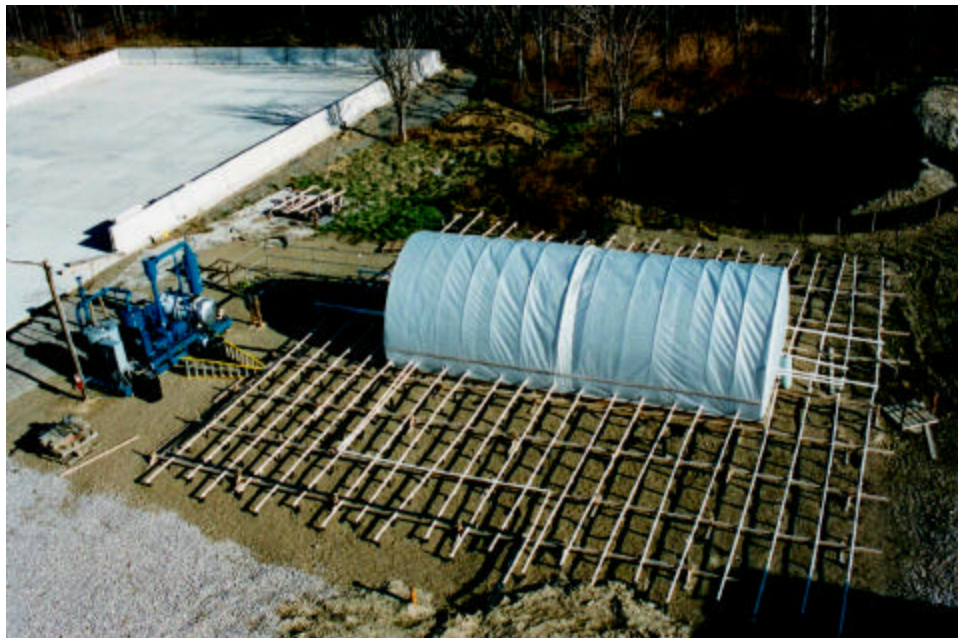
Figure 1. WIDE™ demonstration system.
