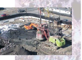
MGP byproducts including DNAPLs and LNAPLs treated in-situ with cement-based S/S.
