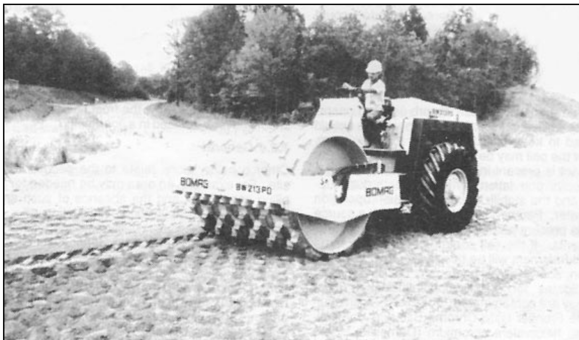
Figure 7-8. Photograph of a sheepsfoot roller being used for compaction.
