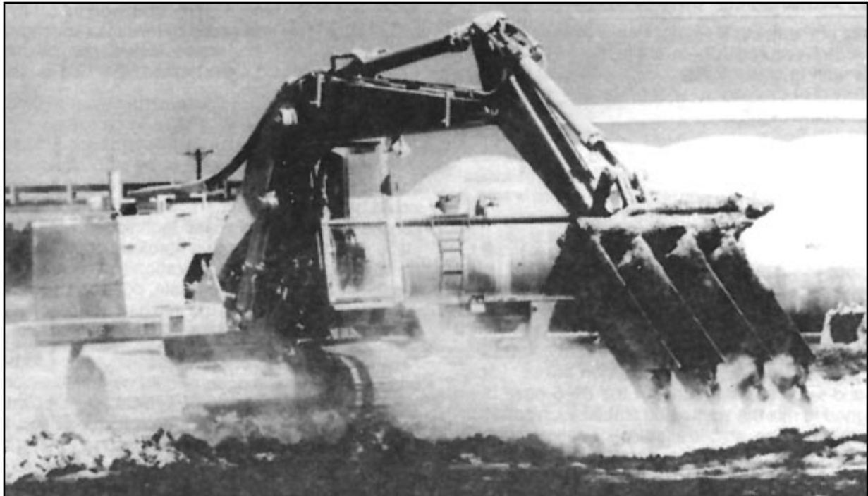
Figure 7-7. Photograph of ENRECO backhoe equipped with stabilization/solidifying agent injector.
