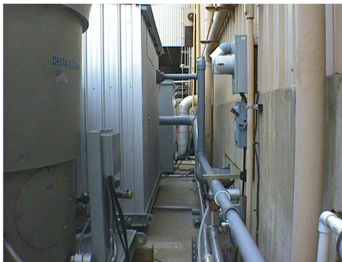
**Figure 3-12. SVE Header Entering Condenser Skid**
