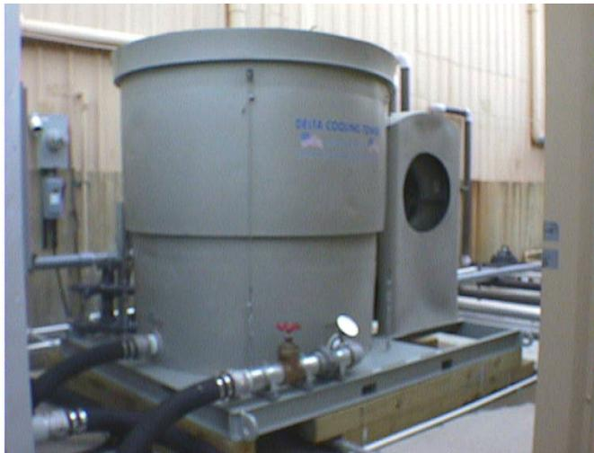
**Figure 3-14. Condenser Cooling Tower**
