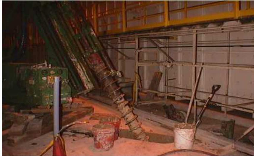
**Figure 3-8. Installation of Angled Electrodes**
