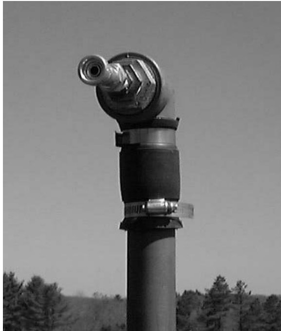
Figure 7.13 Close-up of quick-connect at top of 3.2 cm i.d., sch-80 PVC pipe to prevent gas pressure release at shut-in
