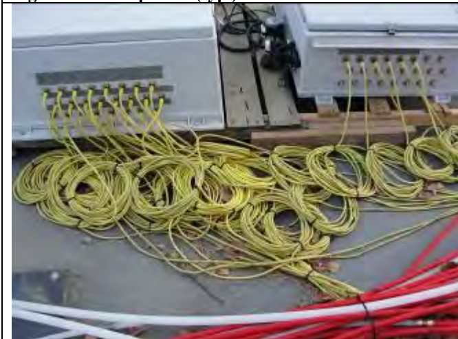
Figure 23 - H2O control panels
