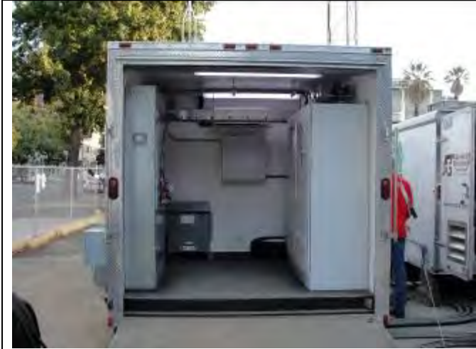
Figure 13 - Feeder switchgear and SCR cabinet with separately derived power
