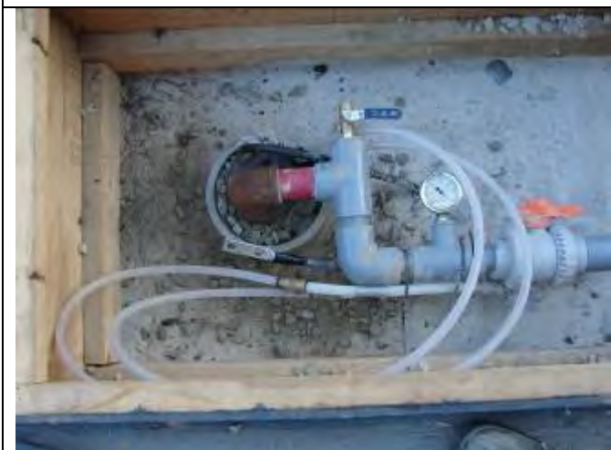
Figure 5 - Well heat with heating cable disconnected, water and pressure manifold (typ.)
