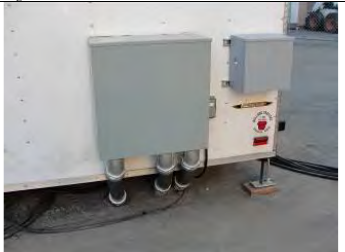
Figure 12 - Feeder terminal enclosure from service
