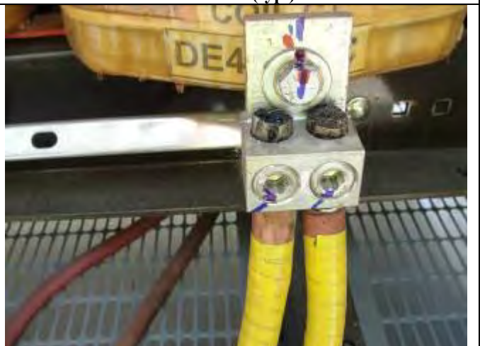
Photo 6 - Connection to terminals (typ.)
