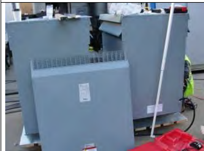
Figure 25 - 480 volt isolation transformers for heating circuits
