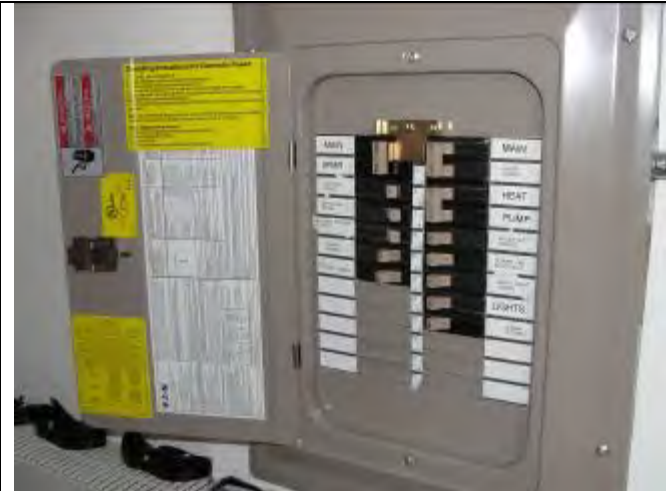
Figure 39 - Trailer sub-panel
