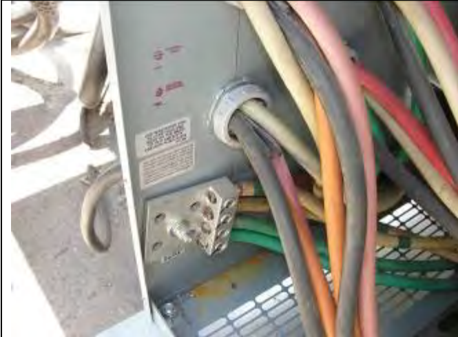
Photo 7 - EGC terminal point (typ.)
