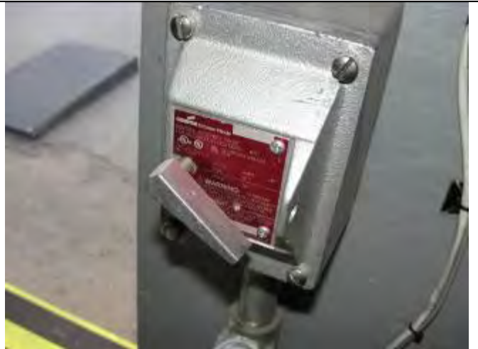
Figure 22 - Disconnect for pump in condensate trailer
