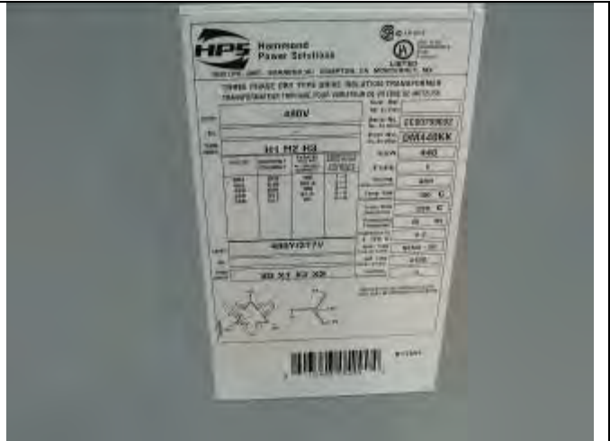
Photo 2 - Transformer 1 label
