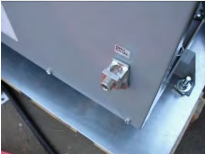
Figure 29 - External bonding connection for bonding two transformer enclosures together
