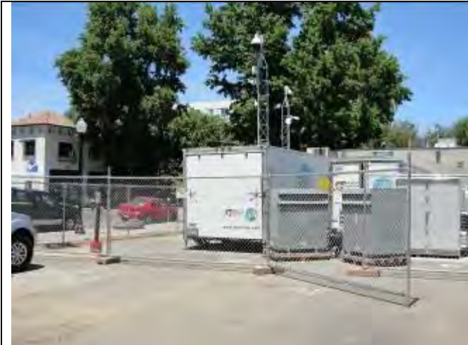
Photo 1 - Site location and new transformers
