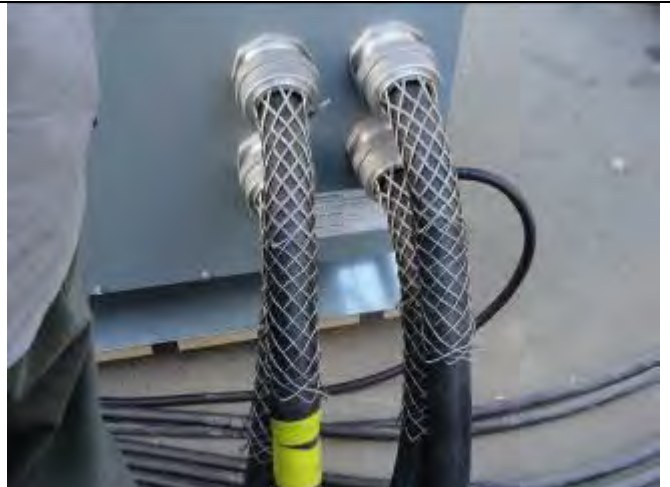
Figure 32 - Termination to transformers of branch circuits (typ)
