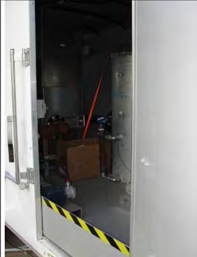
Figure 17 - Inside of condensate trailer
