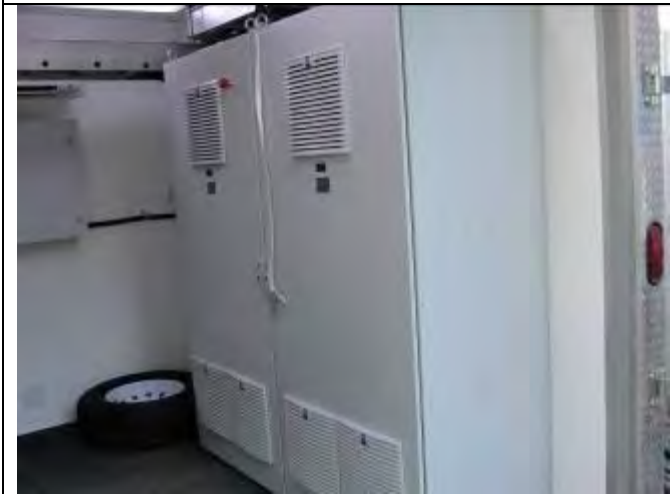
Figure 15 - SCR control enclosures. (two enclosures)
