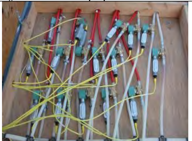
Figure 24 - Control valves enclosure for water injection to wells
