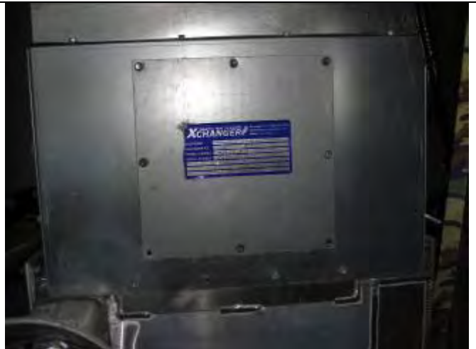
Figure 30 - Nameplate on heat exchanger (typ.)
