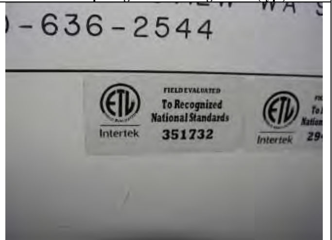
Photo 10 - New field label for transformers only
