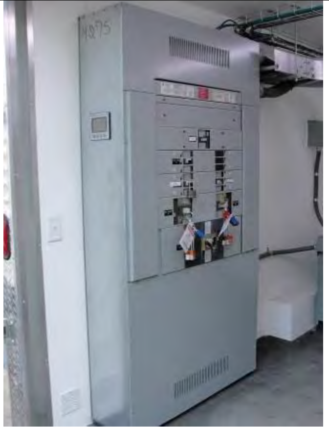
Figure 14 - Feeder switchgear
