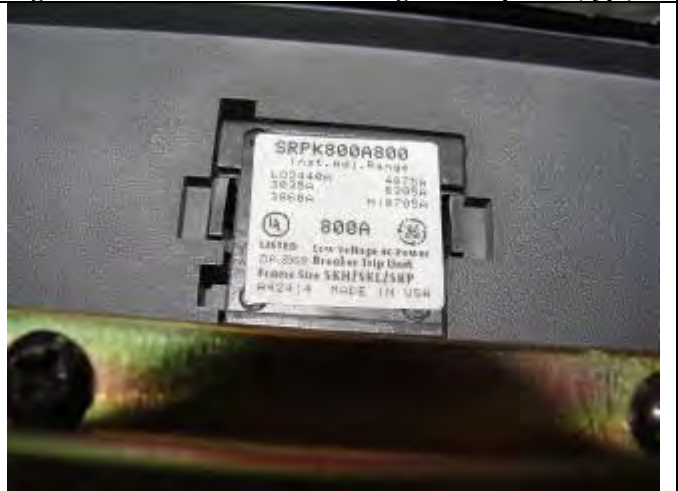
Figure 52 - Ampere rating and fuse plug at feeder panel
