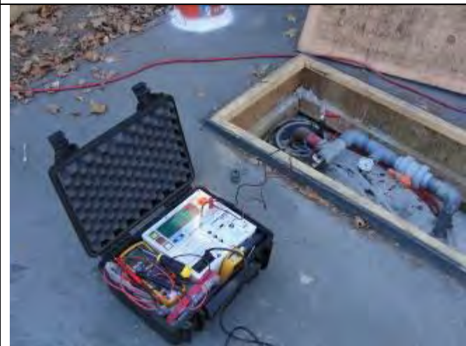
Figure 41 - Dielectric test set up at well head
