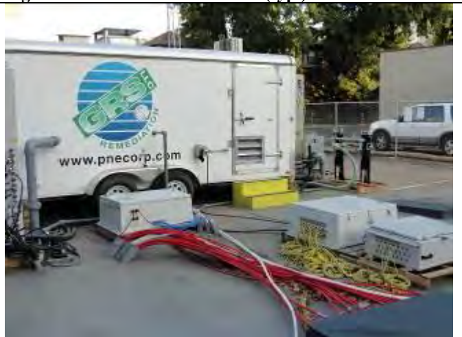
Figure 4 - Condenser trailer with H2O 1 and 2 and TMP control panels
