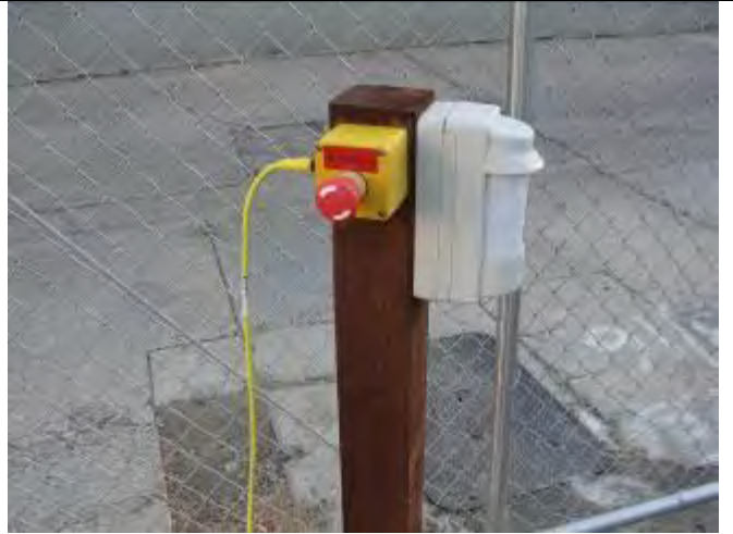
Figure 8 - E-Stop with motion safety sensor (typ.)
