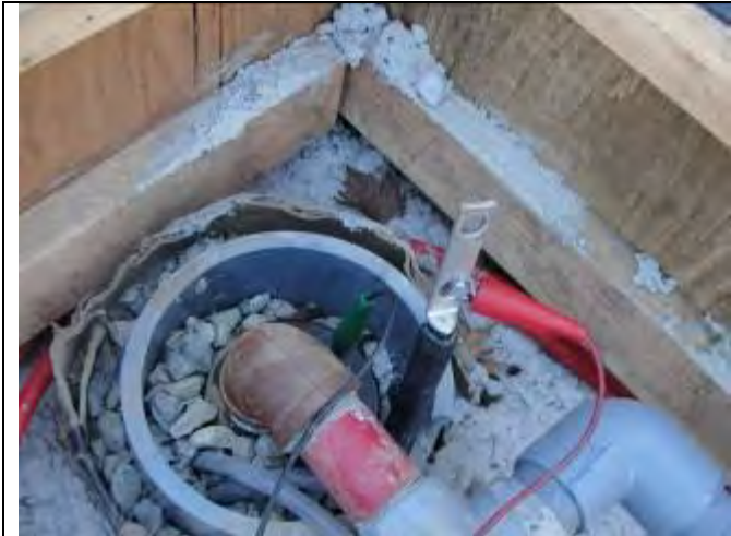
Figure 43 - Conductor under test (typ.)
