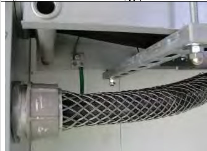
Figure 45 - Cable tray bonding
