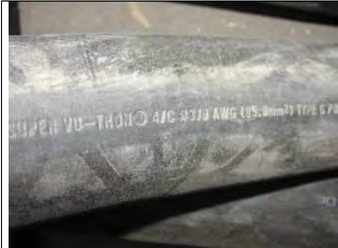
Figure 33 - SOW cables from PDS trailer to transformers and panel EDB-1 (typ.)
