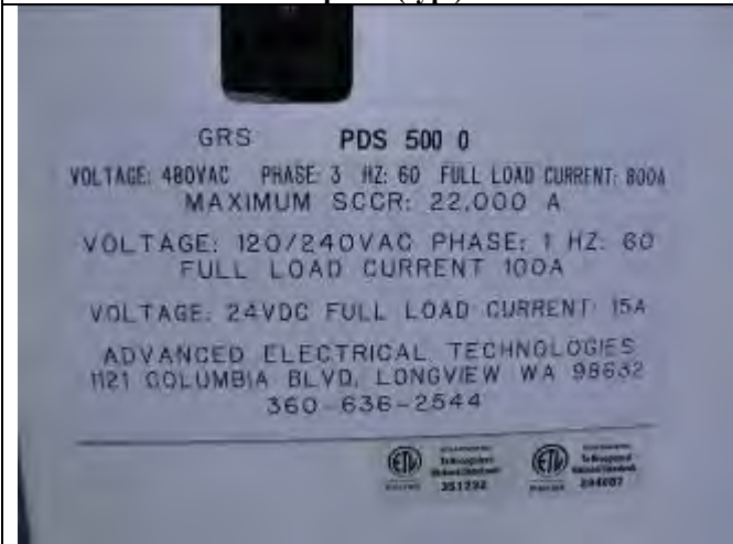
Photo 9 - Nameplate in trailer and ETL field labels
