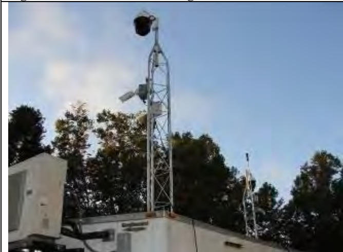
Figure 11 - Security monitoring tower on trailer
