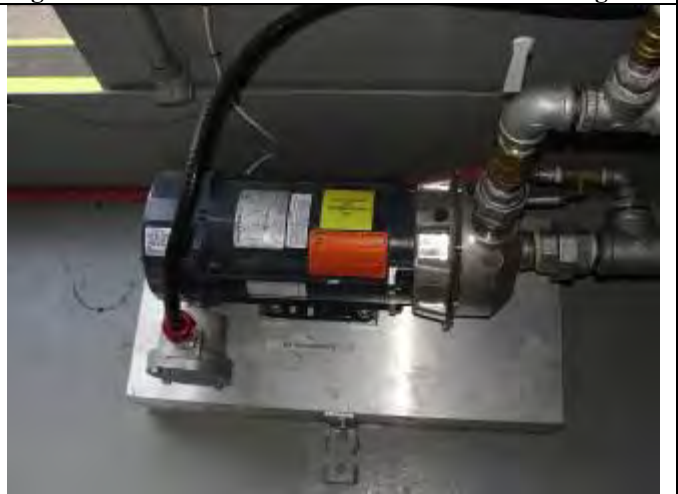
Figure 20 - Effluent pump in condensate trailer
