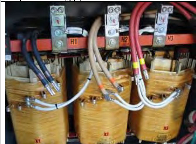
Figure 35 - Transformers with ferrules applied to fine strand conductor (typ.)
