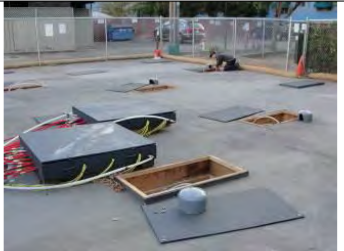
Figure 2 - Well heads and covers (typ.)
