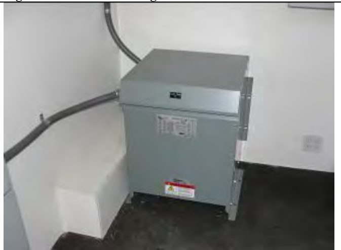
Figure 16 - Separately derived transformer for trailer power
