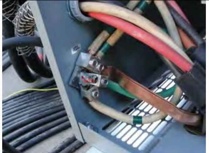
Figure 28 - EGC bonding and termination point
