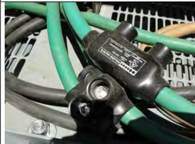
Photo 5 - Spliced equipment grounding conductors (typ.)
