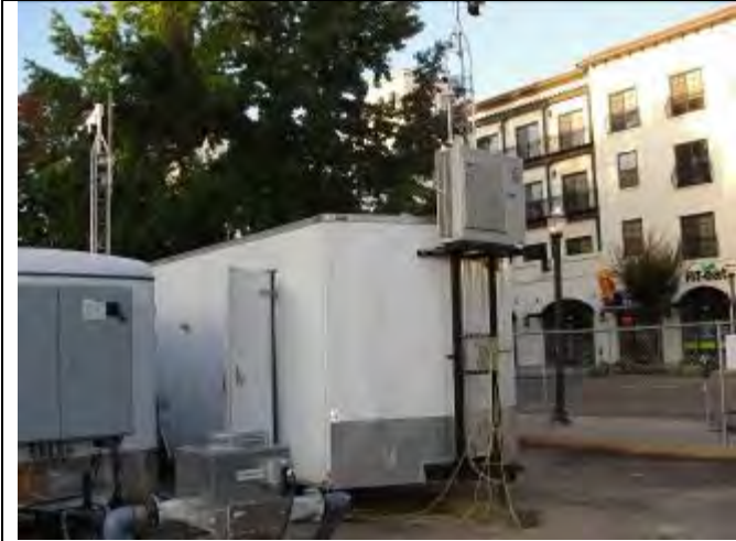
Figure 7 - Power Distribution trailer with security and A/C unit and instrumentation connections
