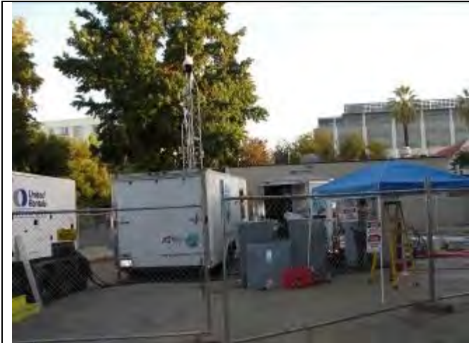
Figure 1 - Site setup with trailers and transformers
