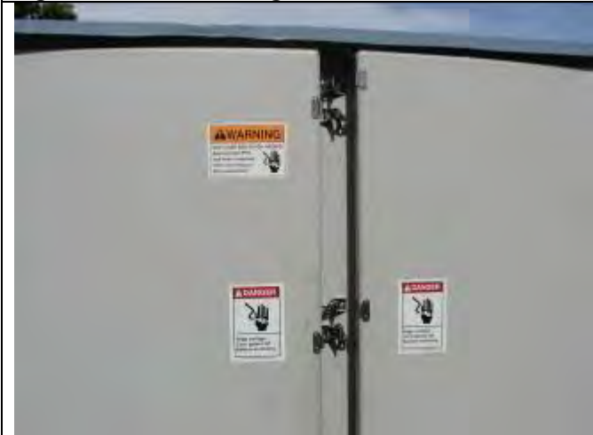
Figure 53 - Warning labels and drip edge modification to panel EDB-1
