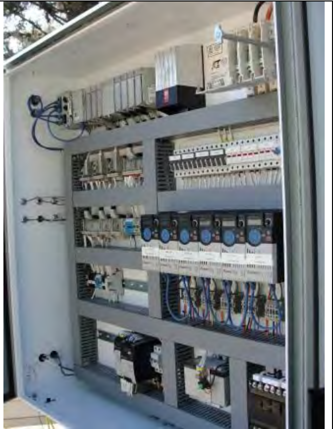
Figure 40 - Condensate trailer control panel
