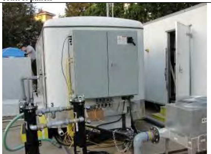
Figure 6 - Condenser control panel with heat exchanger in foreground
