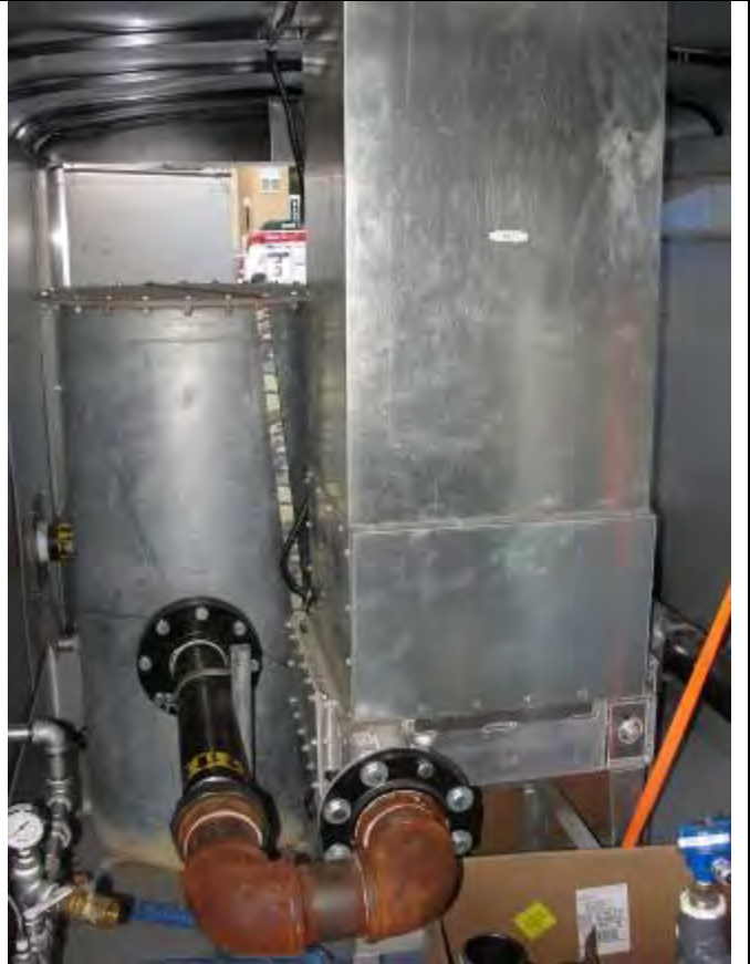
Figure 18 - Condensate tank and inside heat exchanger
