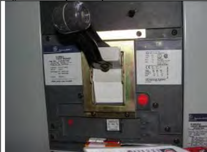
Figure 51 - Feeder switchgear mains
