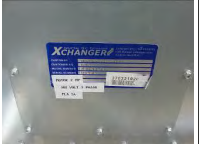
Figure 50 - Corrected heat exchanger nameplates (typ.)
