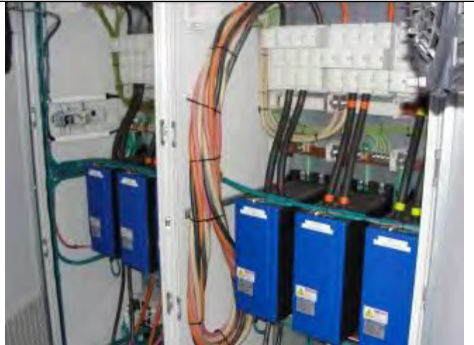
Figure 34 - SCR controllers
