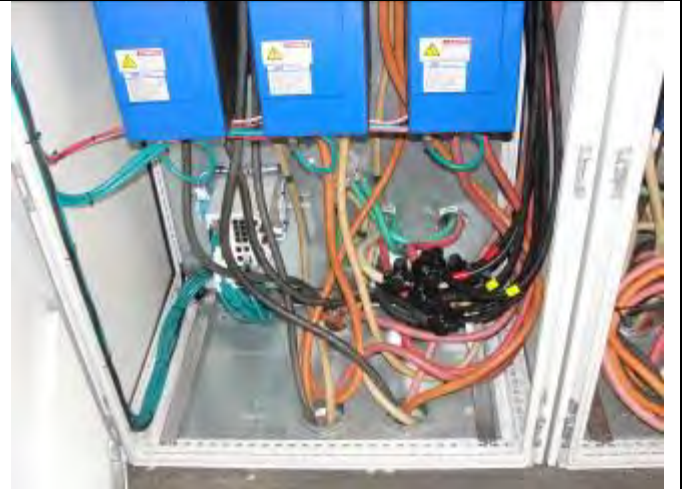
Photo 8 - SCR splicing for new configuration (typ.)
