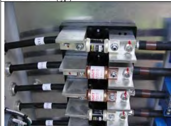
Figure 37 - Conductor termination and fusing for heat lead to sell electrodes (typ.)
