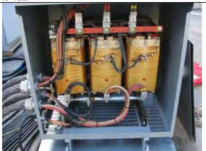
Figure 26 - Interior connection of transformer (typ.)
