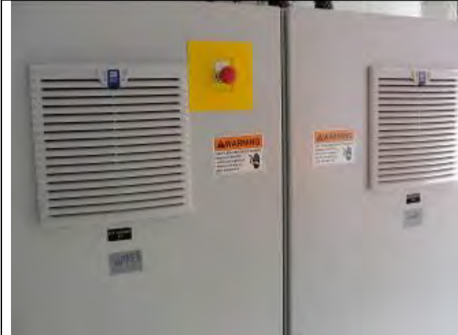
Figure 49 - E-Stop on SCR panel
