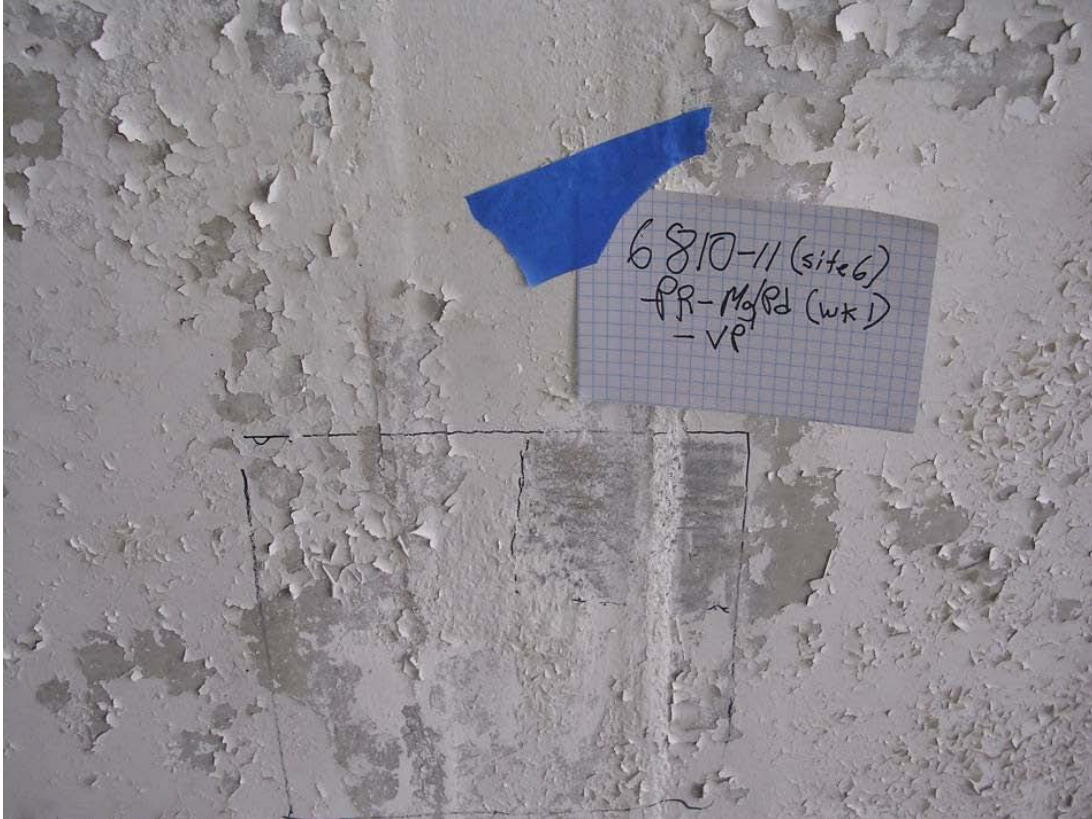
Figure 8. Representative quality of the paint in concrete bunker 6810-11.
