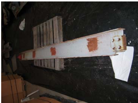
Figure 5-7. Test I-Beam 8 prior to application of BTS
