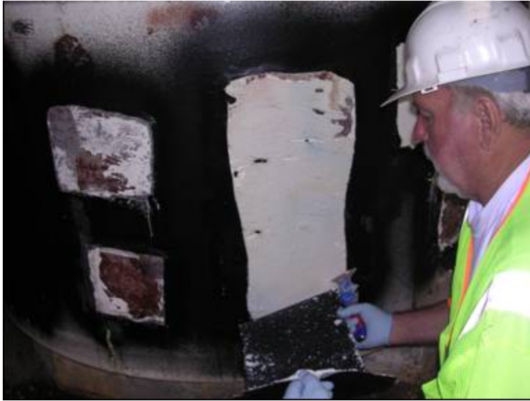
Figure 5-64. Sampling of large tank NM-VP, three weeks after application.
