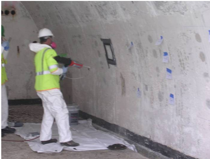
Figure 5-12. Spraying BTS with cartridge-type spray gun.
