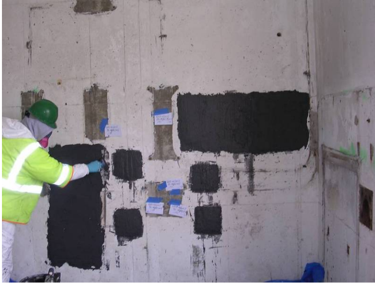
Figure 5-18. Application of Mg/Pd BTS prior to sealing with VP or silicon sealant, 6810-36.
