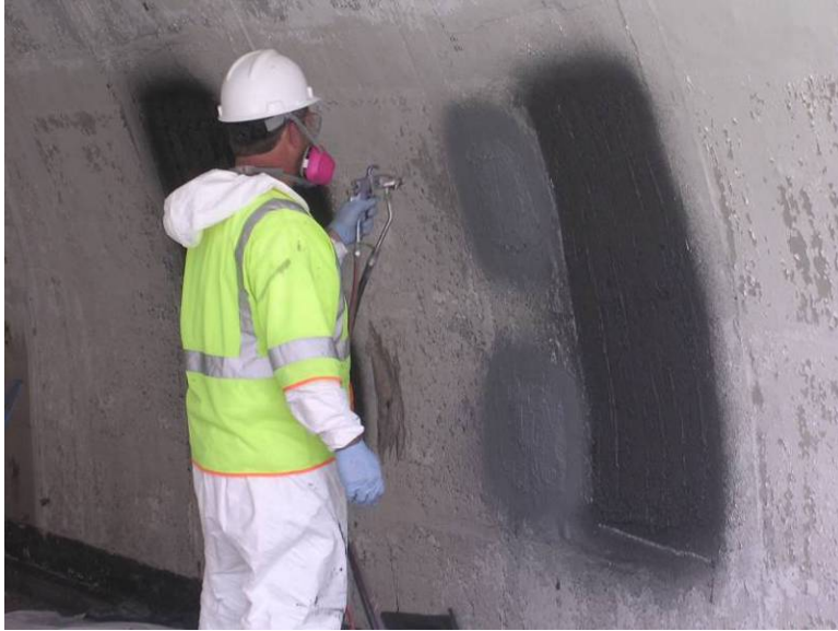
Figure 5-14. Silicon sealant application with spray gun.
