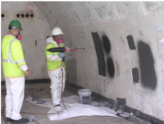
Figure 5-13. Vinyl polymer sealant application using cartridge spray gun.
