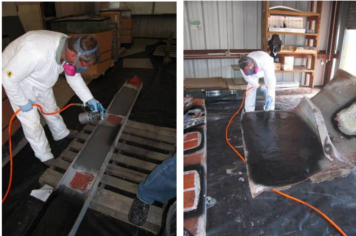
Figure 5-11. Application of coating material using HVLP sprayer.
