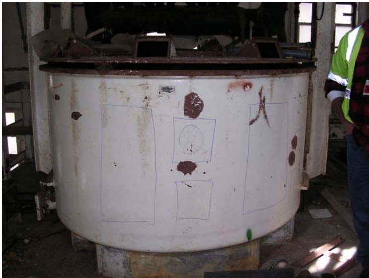
Figure 5-84. Quality of the paint on the tanks in the nitrating house.
