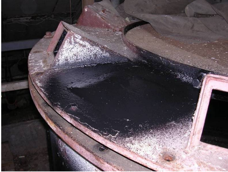
Figure 5-25. Large tank lid, treated with Mg/Pd-VP, immediately after application.
