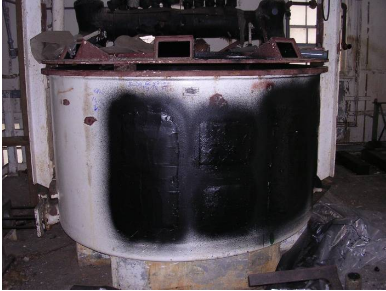
Figure 5-23. Large tank treated with Mg/Pd-VP and NM-VP immediately after application – view 1.
