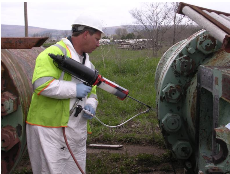
Figure 5-29. Vinyl polymer (VP) sealant being applied to press 15.
