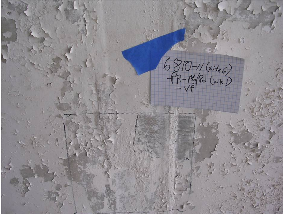
Figure 5-83. Representative quality of the paint in concrete bunker 6810-11.
