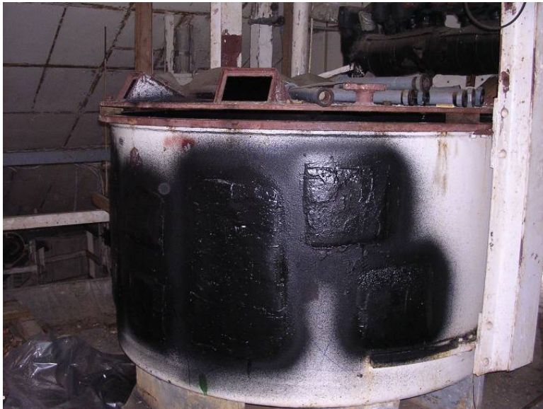
Figure 5-24. Large tank treated with Mg/Pd-VP and NM-VP immediately after application - view 2.
