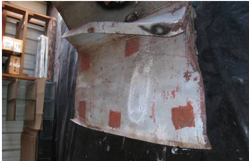
Figure 5-6. Test Panel 4 prior to application of BTS
