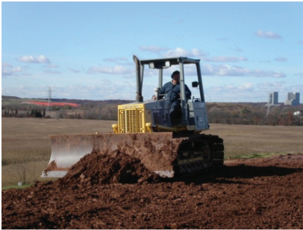
Placing clay on landfill
