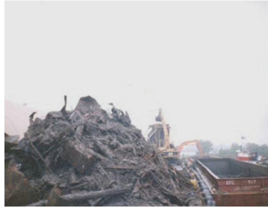
Debris pile from harbor job
