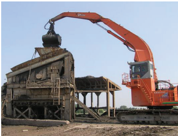
Stacked vibratory screens
