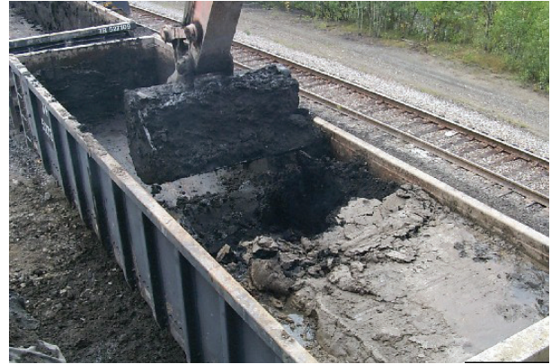
Unloading PDM from rail car
