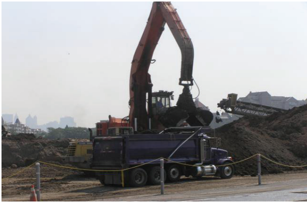
Loading of PDM into truck
