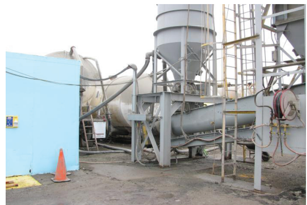
Pneumatic pozzolan metering system
