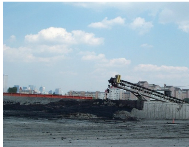
Radial stacker and PDM containment area
