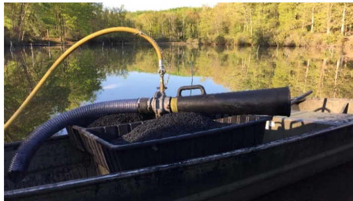
Figure 29. Modified VHI Utilizes a Vacuum Generated by Compressed Air through a Venturi to Propel SediMite to the Desired Area.
