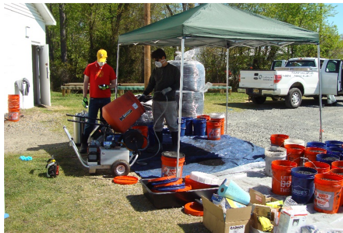
Figure 33. Staging Area at Abrahams Creek Used to Prepare Bioamended SediMite Prior to Deployment.
