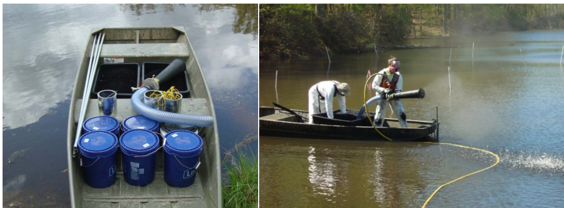
Figure 34. Flat Bottom Boat Loaded with VHI System, Hoppers Filled with Bioamended SediMite and 20 L Buckets of Bioamended SediMite for Refilling Hoppers (left panel); Application of Bioamended SediMite™ at Abraham's Creek (right)
