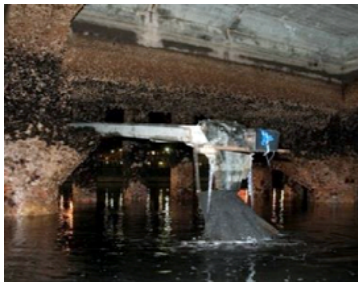
Figure 13. Reactive Amendment Placement beneath Pier (via Conveyor) at BNC Study Site (Courtesy of ESTCP)
