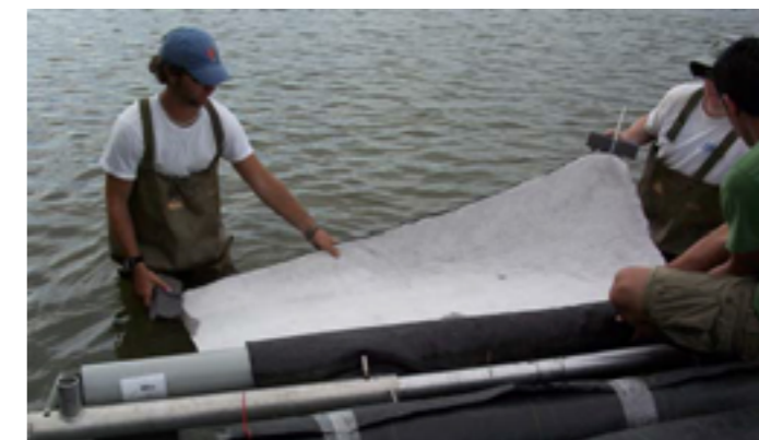
Figure 11. Small-scale geotextile test mat deployment.
