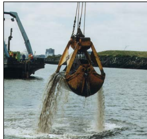
The grab appears to have fully closed but there is still significant release of material due to spillage from the top of the grab.
