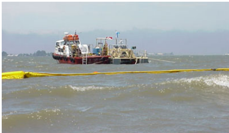
Figure 7. Floating curtain deployed in San Francisco Bay (courtesy of Julie Kistle, KFM-Joint Venture, San Francisco-Oakland Bay Bridge East Span Skyway Project Turbidity Monitoring Project)
