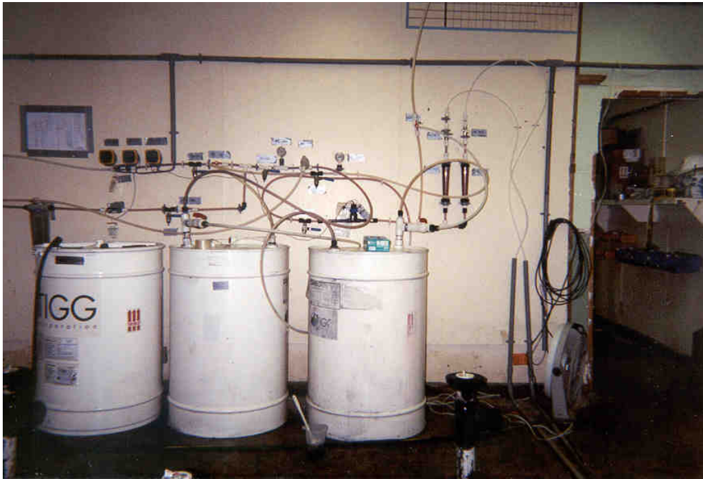
Figure 3-4. Aboveground Water Treatment System (A Series of Two Carbon Tanks and a Backup Tank)
