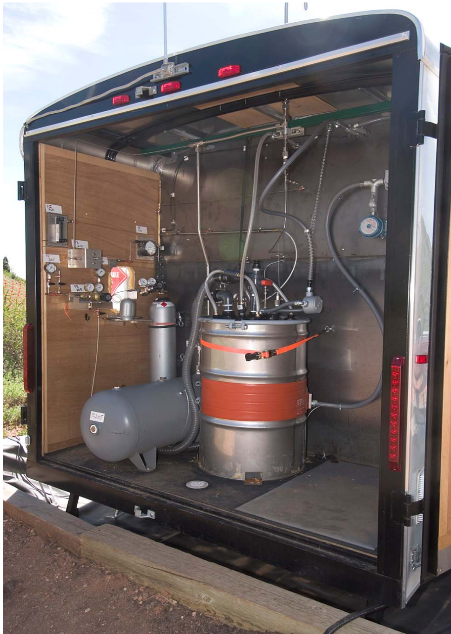
Hydrogen component side of treatment trailer, showing nickel catalyst reactor with stainless-steel drum (May 2006).
