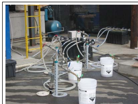
Figure 1. ISCO Application Wells
