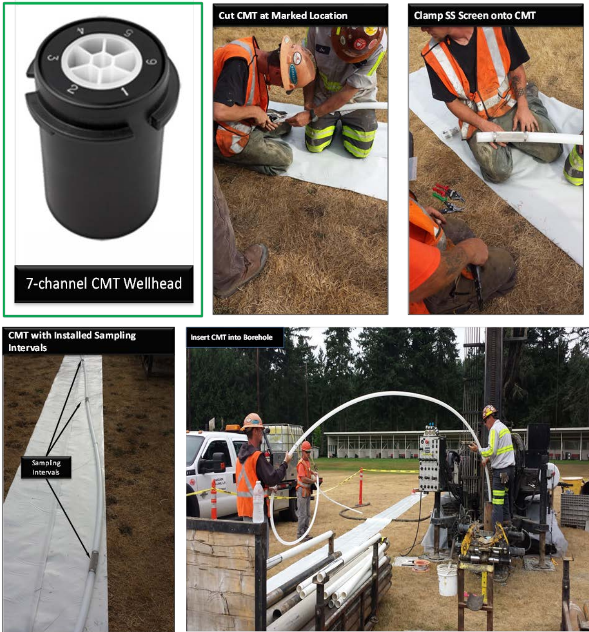
Figure 5.10. CMT well installation during field demonstration. Photos illustrate several key steps (not all steps shown).
