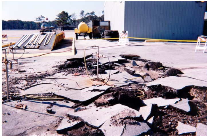
Figure 3-2. Rupture of asphalt due to rapid pressure release during injection of 25% H 2 O 2
