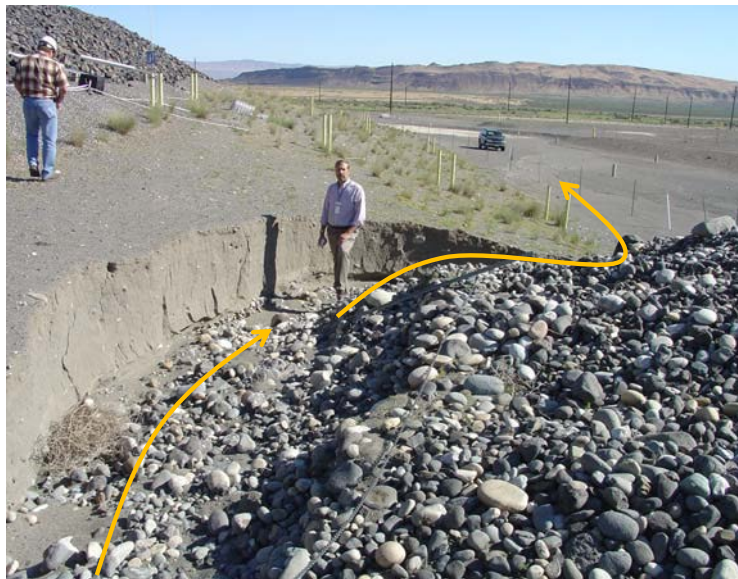
Figure B.11. North-facing photograph taken on June 16, 2004. The orange lines indicate the path and direction of the runoff.
