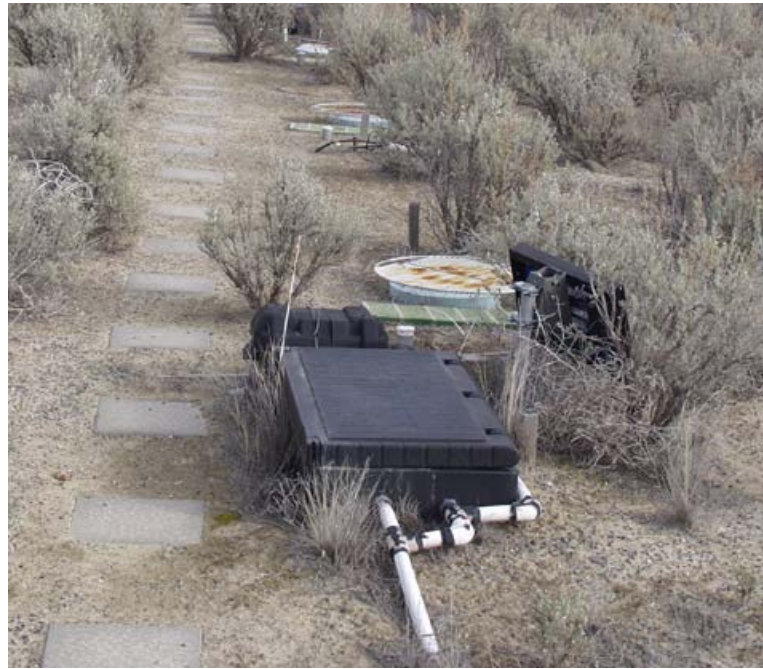
Figure C.15. The conduits for wires and enclosure for the dataloggers and barriers.
