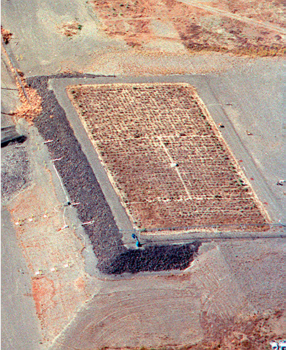
Figure O.5. The Prototype Hanford Barrier on June 2, 1999 (southwest-facing view).
