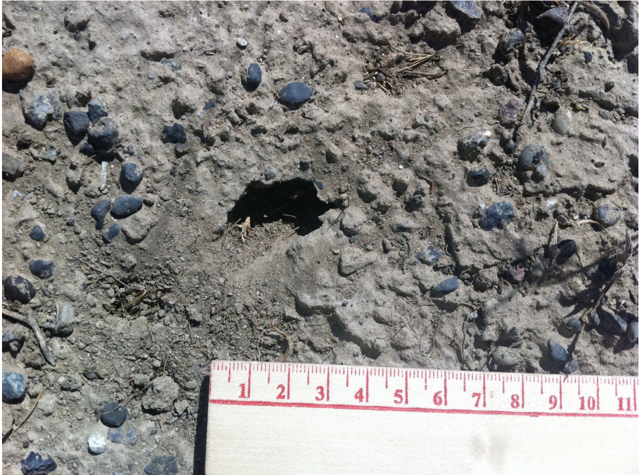
Figure L.5. Small Animal Hole on the Burned Section of the Barrier Surface.
