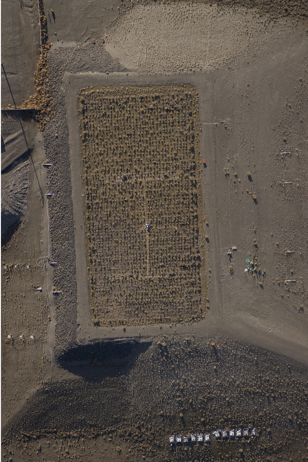
Figure O.7. The Prototype Hanford Barrier on January 3, 2003 (southwest-facing view).
