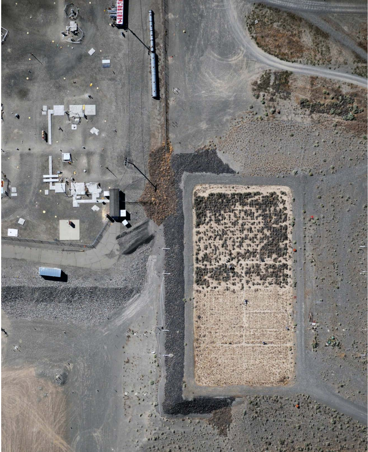
Figure O.11. The Prototype Hanford Barrier on August 18, 2011 (south-facing view).
