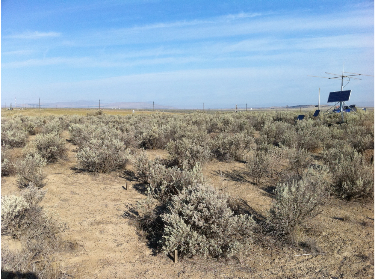
Figure J.7. Prototype Hanford Barrier cover dominated by Artemisia tridentata in 2010, 16 years after establishment on the unburned section of the surface.
