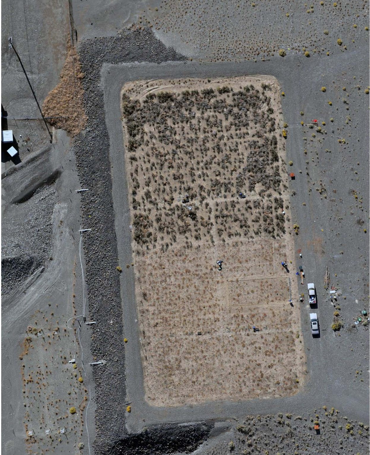
Figure O.10. The Prototype Hanford Barrier on September 30, 2009, 1 year after the controlled burn (south-facing view). The north half was still mostly free of vegetation.
