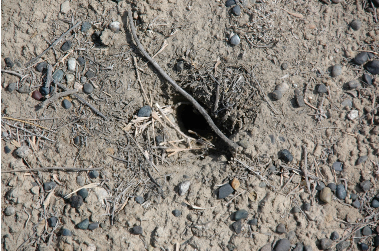
Figure L.4. Typical Animal Hole on the Surface of the Barrier.
