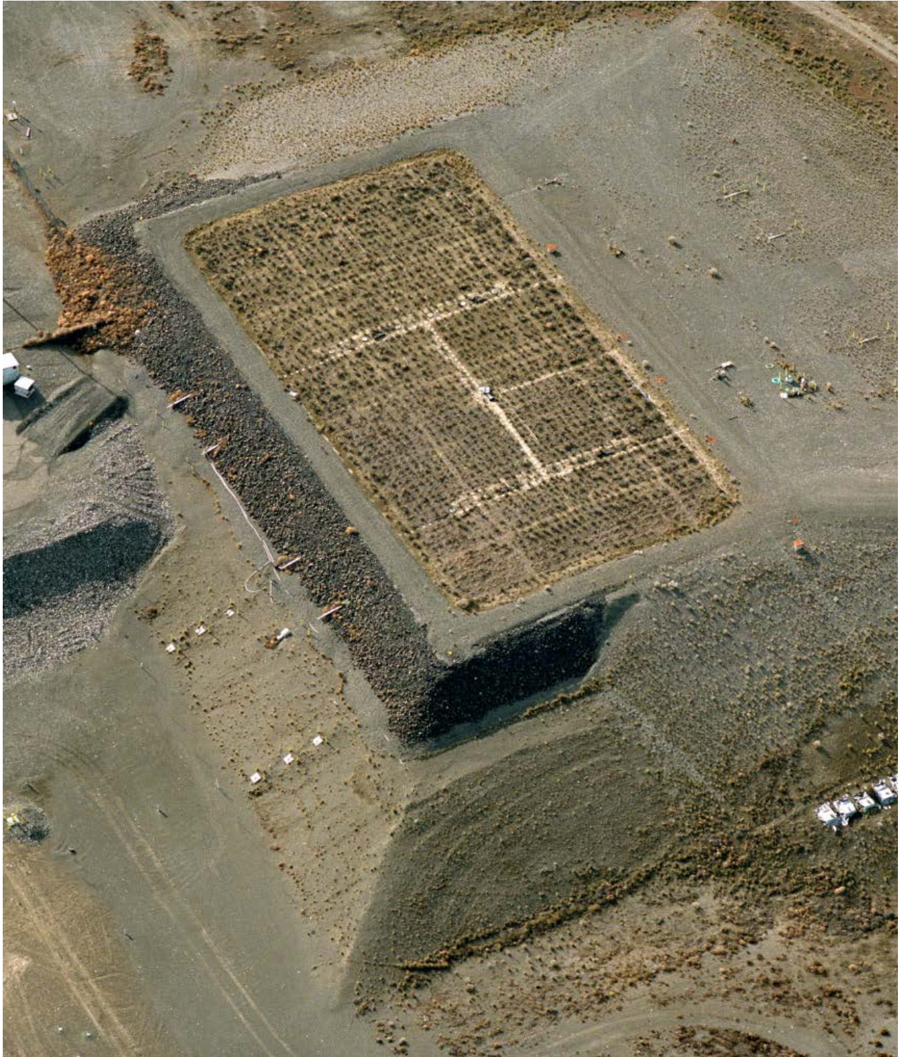
Figure O.6. The Prototype Hanford Barrier on September 17, 2002 (southwest-facing view).
