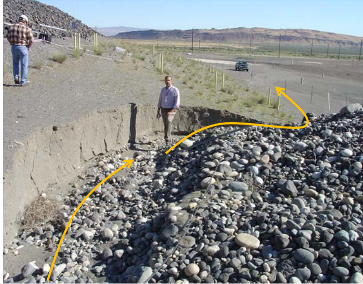
Figure I.9. North-facing photograph taken on June 16, 2004. The orange lines indicate the path and direction of the runoff water in May 2004 after severe thunderstorms.
