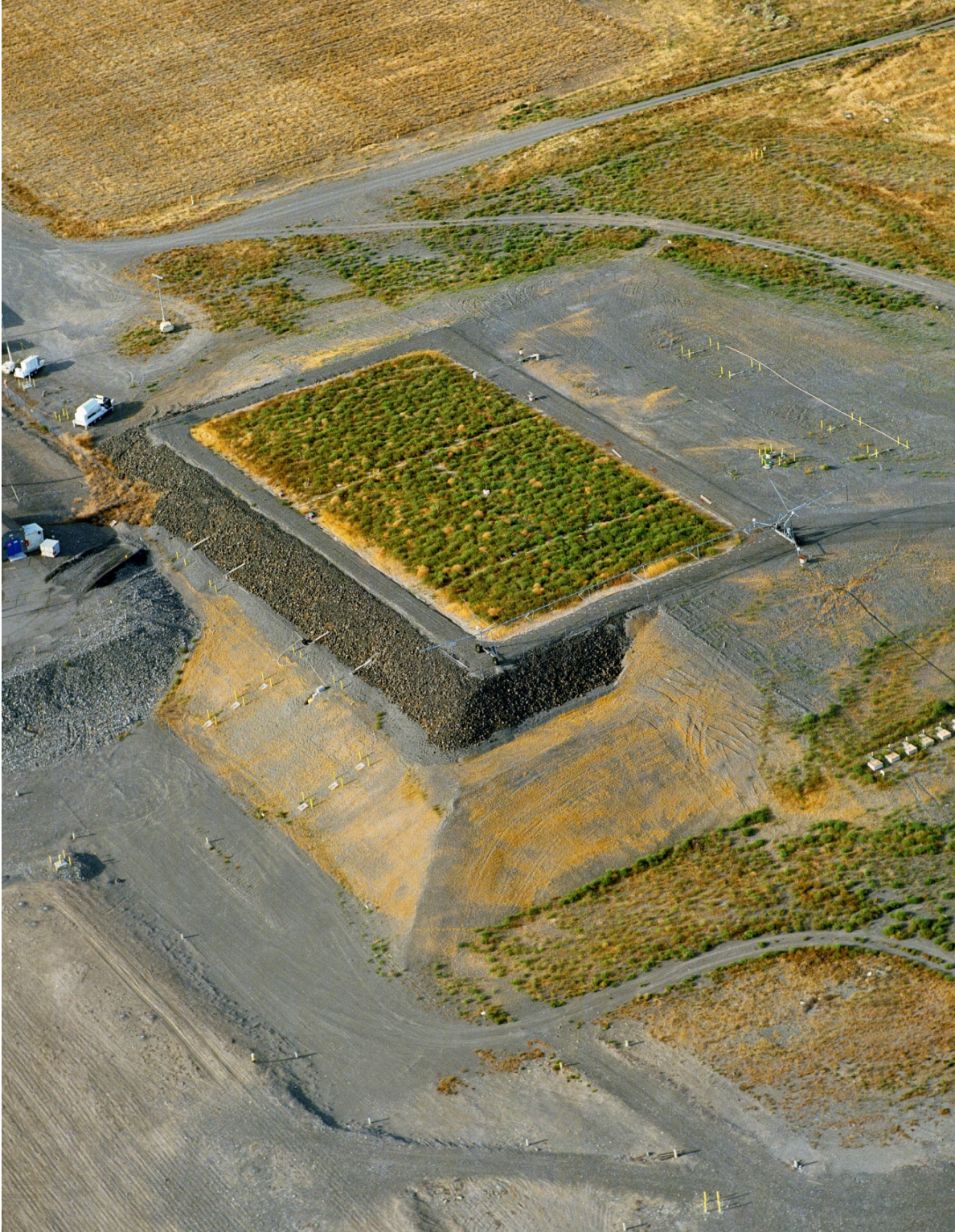
Figure O.2. The Prototype Hanford Barrier on August 9, 1995 (southwest-facing view). The green vegetation seen in the photo is non-native Russian thistle (tumbleweeds), not the planted native sagebrush and rabbitbrush, which were still seedlings and were much smaller than the Russian thistle, and cannot be seen in the image. The Russian thistle might come with the imported silt loam.
