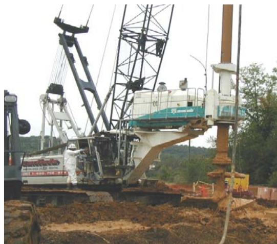
Figure 6-7. ZVI-clay application using soil mixing.
