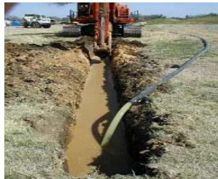
Figure 6-4. Biopolymer trench construction.
