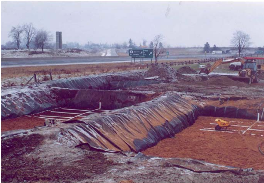
Figure 6-1. Horizontal PRB for treatment of septic system nitrate. (Courtesy of Septech, Inc., 2003)
