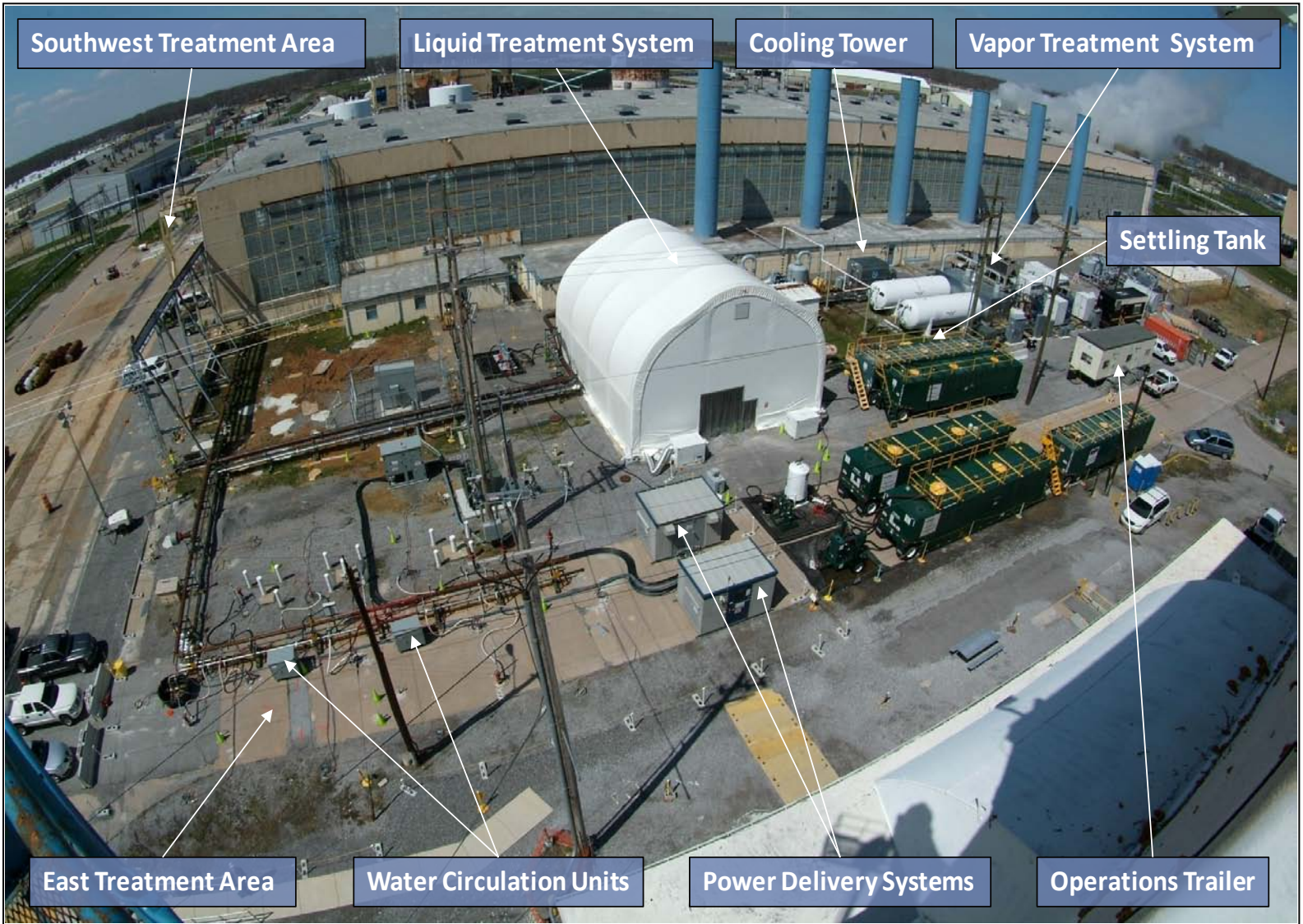
Figure 27. Picture of Groundwater/Vapor Treatment System Area
