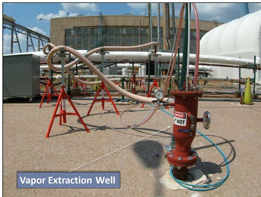
Figure 18. Vapor Extraction Well
