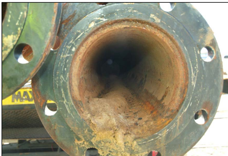
Figure 25. Sediment in the Vapor Extraction Header
