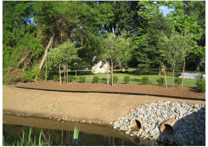
Adjacent Surface Water: Treated water from the offsite plant discharges into the adjacent "Mill Creek," which flows to the Long Island Sound. The creek bank was stabilized by seeding deep-rooted wetland species, covering the seeded areas with jute mat that provides an anchor, and emplacing a layer of erosion-resistant rock around stormwater control culverts.
