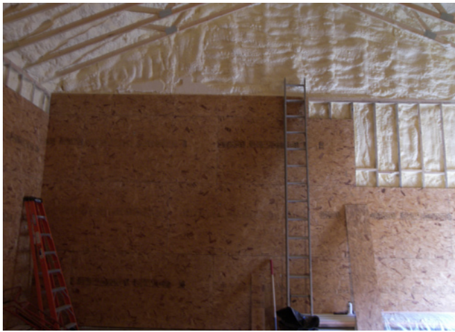
Building Insulation: Construction bids for the offsite treatment building required spray-foam insulation due to its ability to serve as a moisture and dust/pollen barrier and high insulating value, which results in lower energy consumption and HVAC loads. High density of the foam and its tight placement among framing components also helps reduce noise impacts on nearby residential properties.
