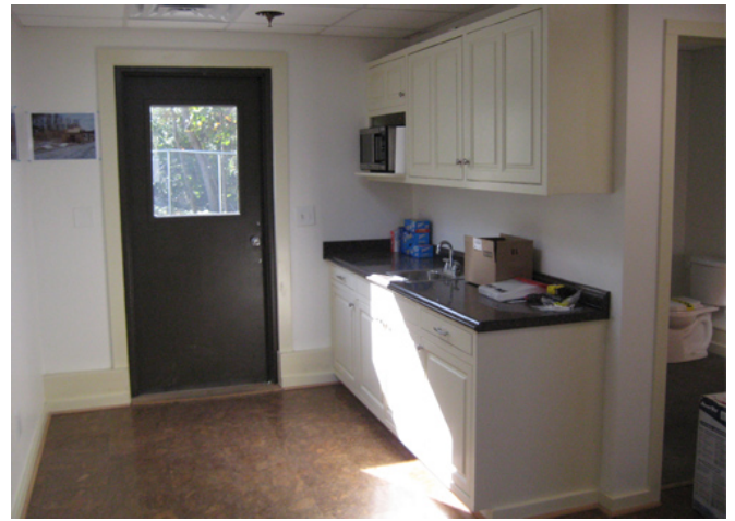
Interior Features: All trim board in the offsite treatment building consists of 72-85% recovered or recycled fiber certified by a third party using Scientific Certification Systems. Cork flooring above a rigid foam layer provides moisture and antimicrobial protection, cushioning, and noise reduction in the break-room, which receives natural daylight by way of a high-efficiency window. Cabinetry or shelving constructed of salvaged framing waste stores routine supplies or processing equipment.
